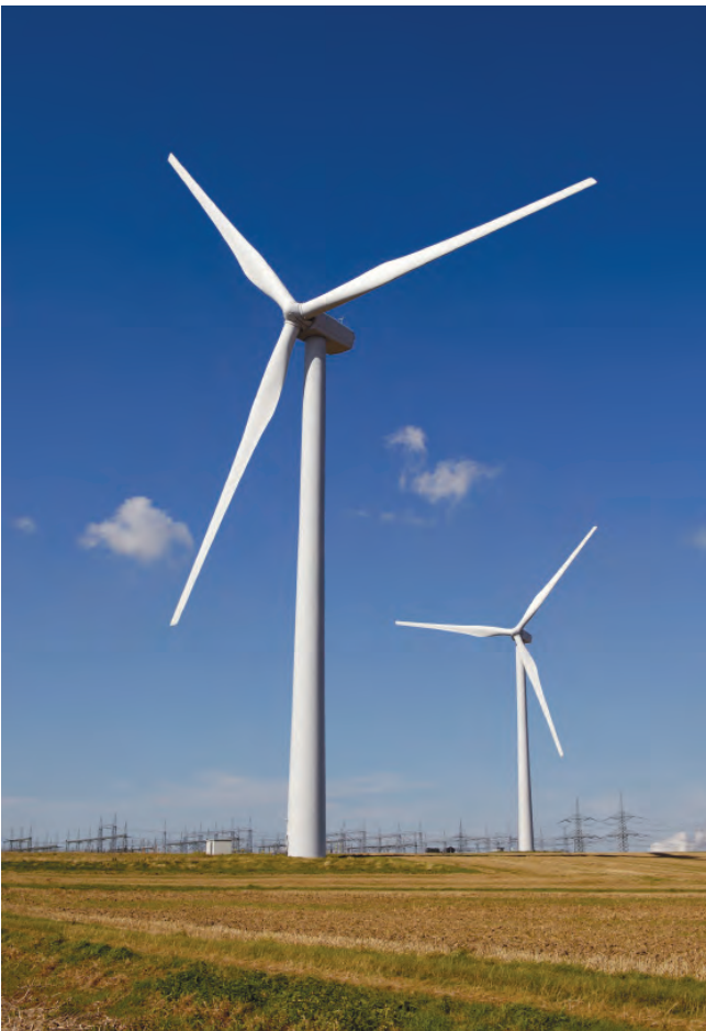
Figure 7. Shielded flexible conduits are specified to address EMI/RFI issues in wind turbine controls as well as solar applications.
